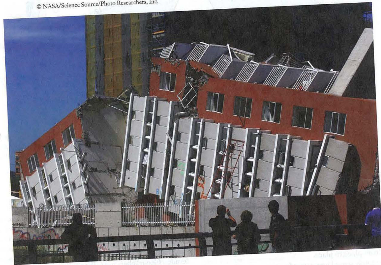
Figure 1.13 Concepcion, Chile. Chile has broadly adopted engineering and architecture practices that lessen the impact of earthquakes. Although the 2010 earthquake caused over $30 billion worth of damage, it could have been much worse without these building practices. Most of the damage in Concepcion was to residential buildings like this one. © AP/Wide World Photos.
